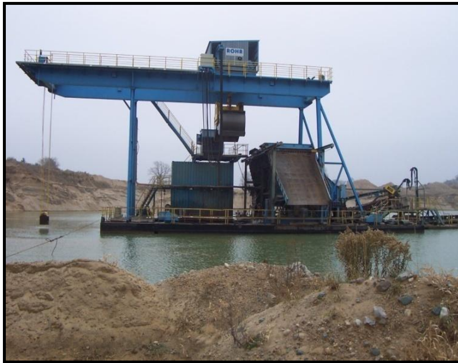
Figure 1.1 Clamshell dredge on site
